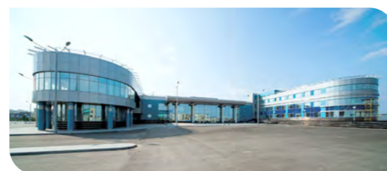
MULTIFUNCTIONAL STATION, NEW URENGOI Commissioned in 2015
