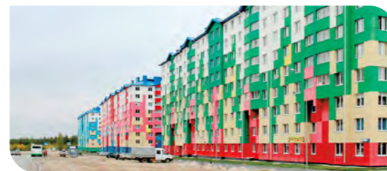
NORTHERN LIGHTS RESIDENTIAL COMPLEX, NOYABRSK Commissioned in 2015
