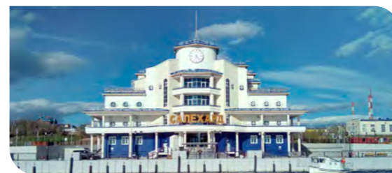
RIVER STATION COMPLEX, SALEKHARD Commissioned in 2015
